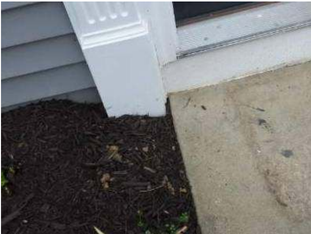
Photo 4-3 Soil in contact with trim.
