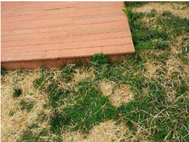
Photo 2-1 Soil in contact with decking structure.
