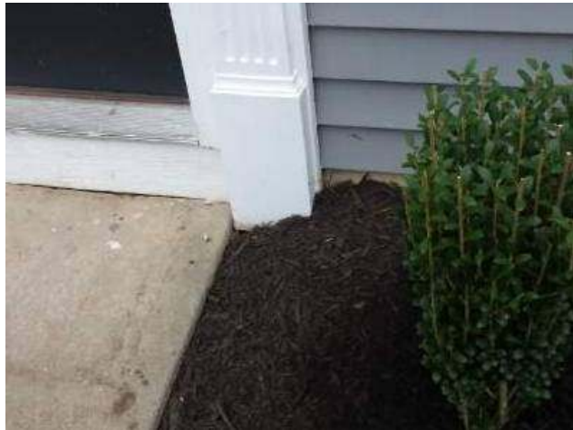
Photo 4-4 Soil in contact with trim.
